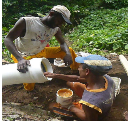
Figure 10 Picture showing Spigot and socket jointing Source: Pelena Energy
