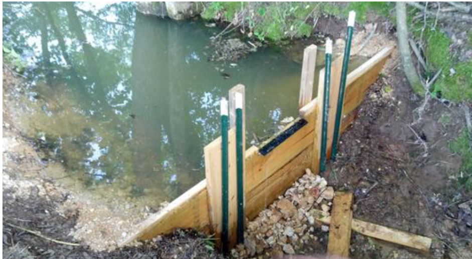
Figure 4 Simple stop-log and rack kind of arrangement Source: Pond Boss magazine
