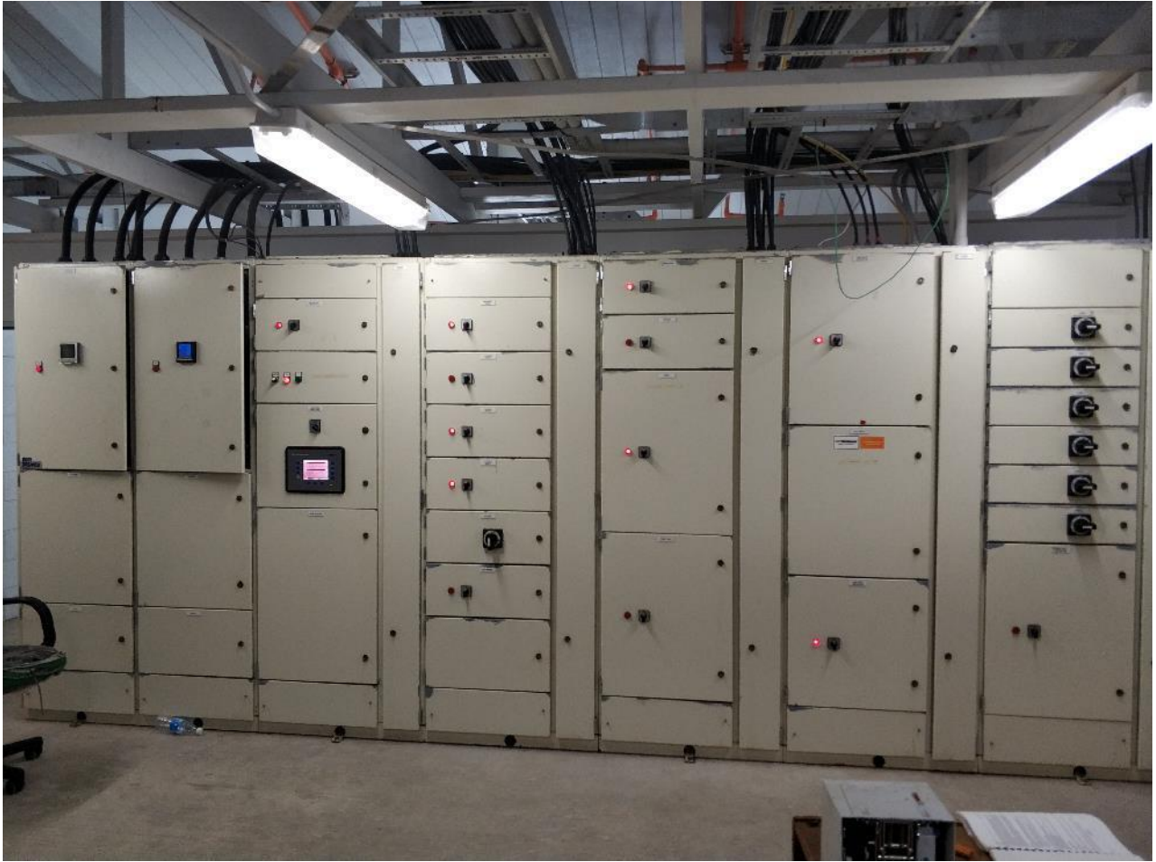
Figure 11: Existing switchboard at CMI
