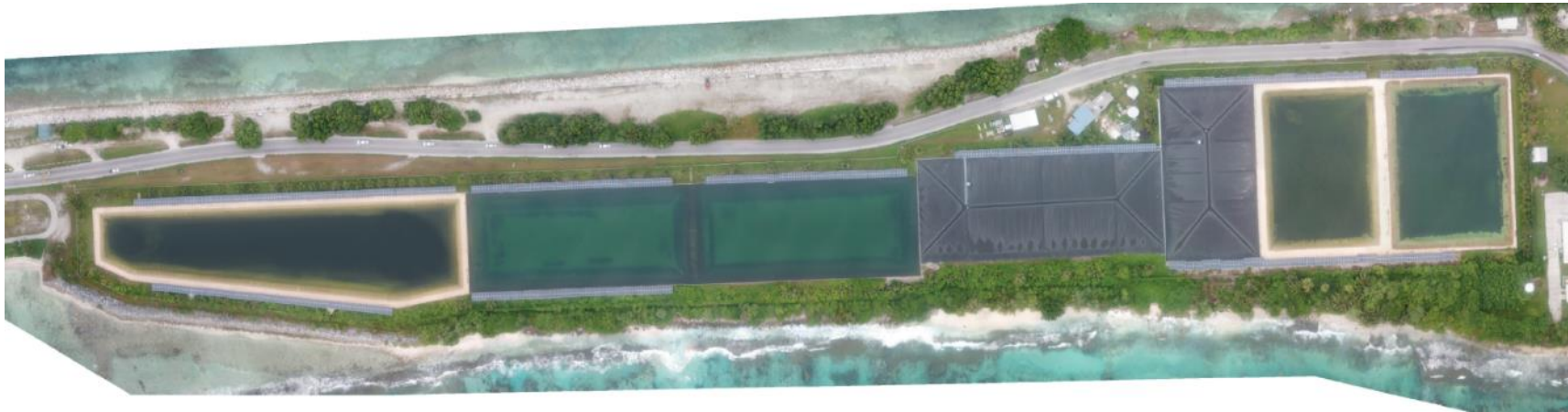
Figure 3: Drone footage of reservoirs showing locations of existing PV arrays
