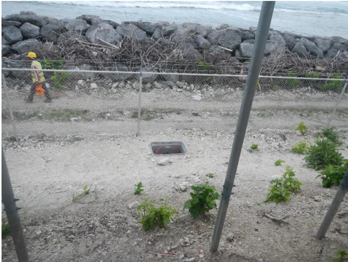
Figure 5: Access track on ocean side of reservoirs and existing solar cable pit. Note, this photo was taken 2 years ago and the track is now overgrown.
