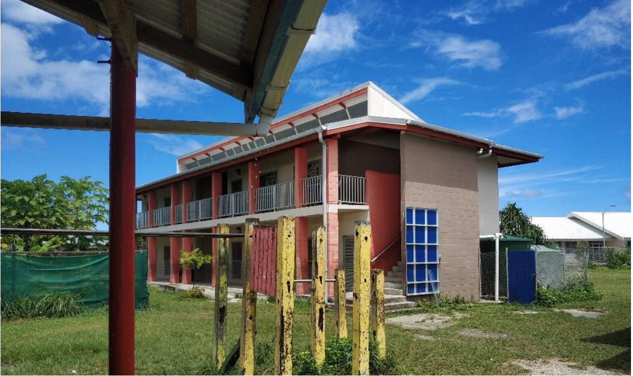
Figure 7: School building at Rita Elementary School
