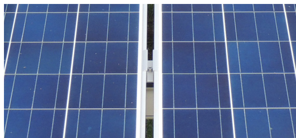
Figure 7: 50mm (2 inch) mid-clamps
