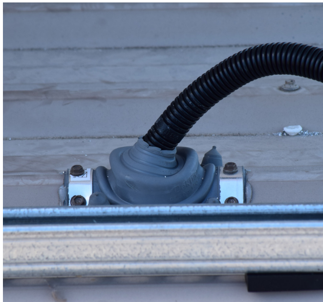
Figure 17: A collar flashing on a metal roof
