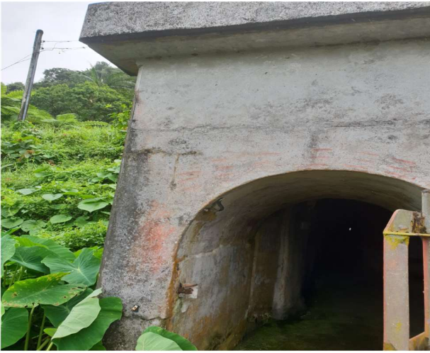
Entrance to Tunnel #2
