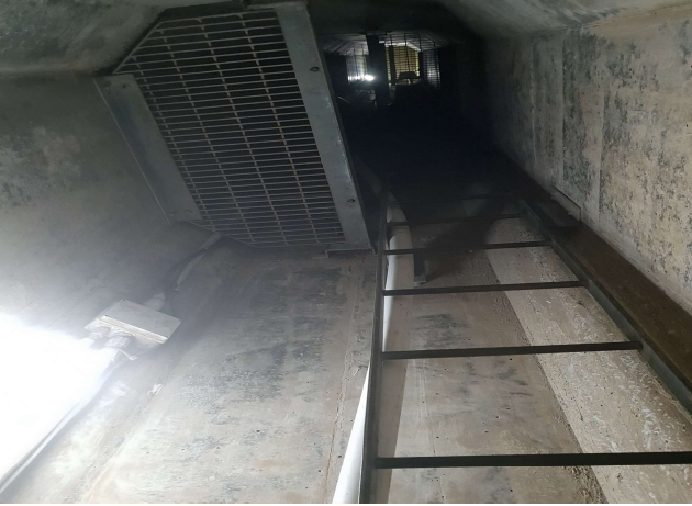
Ladders in Tunnel #1
