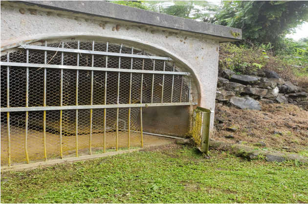
Entrance to Tunnel #1
