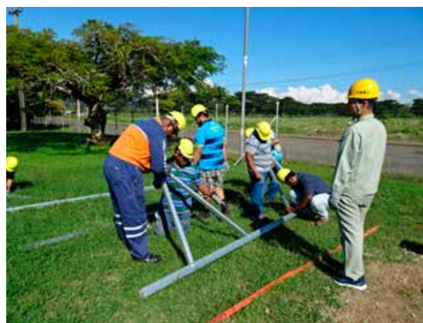
Installation of Training PV system (3.5kW) in Fiji
