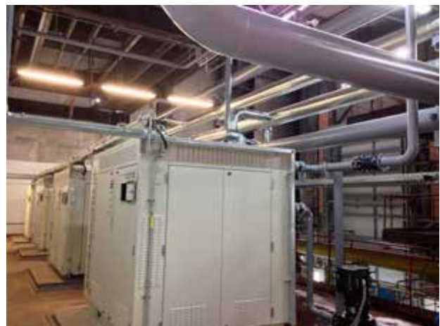
Figure 2. ElectraTherm installed ten POWER+ GENERATOR 4400s at a district heating plant in Slovakia.
