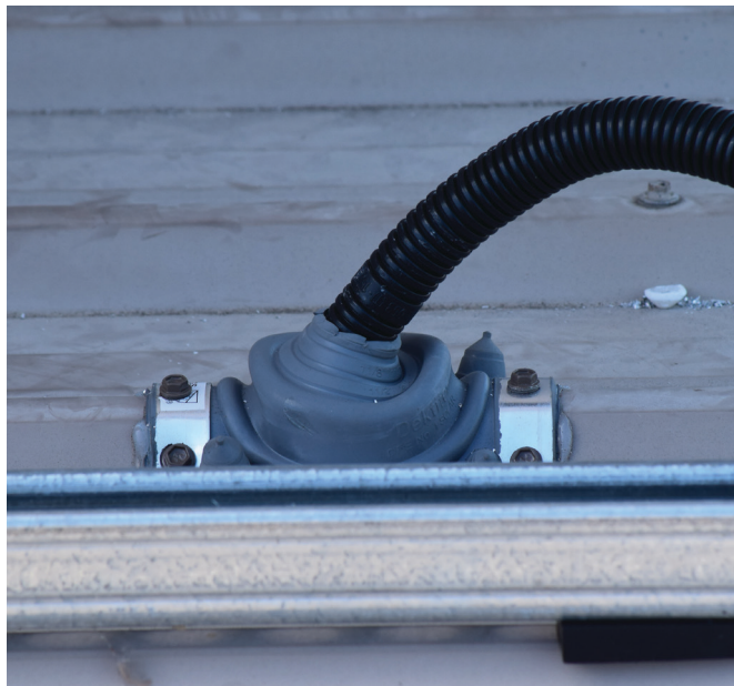
Figure 17: A collar flashing on a metal roof
