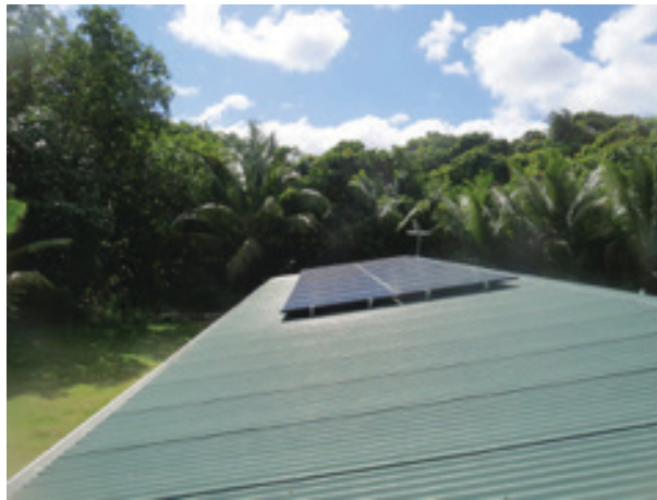
Figure 6: Array on House Roof
