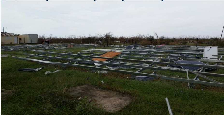
Solar plant completely destroyed
