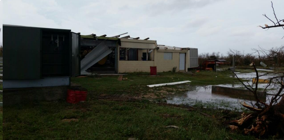
Damaged roof of power plant that houses the Generators
