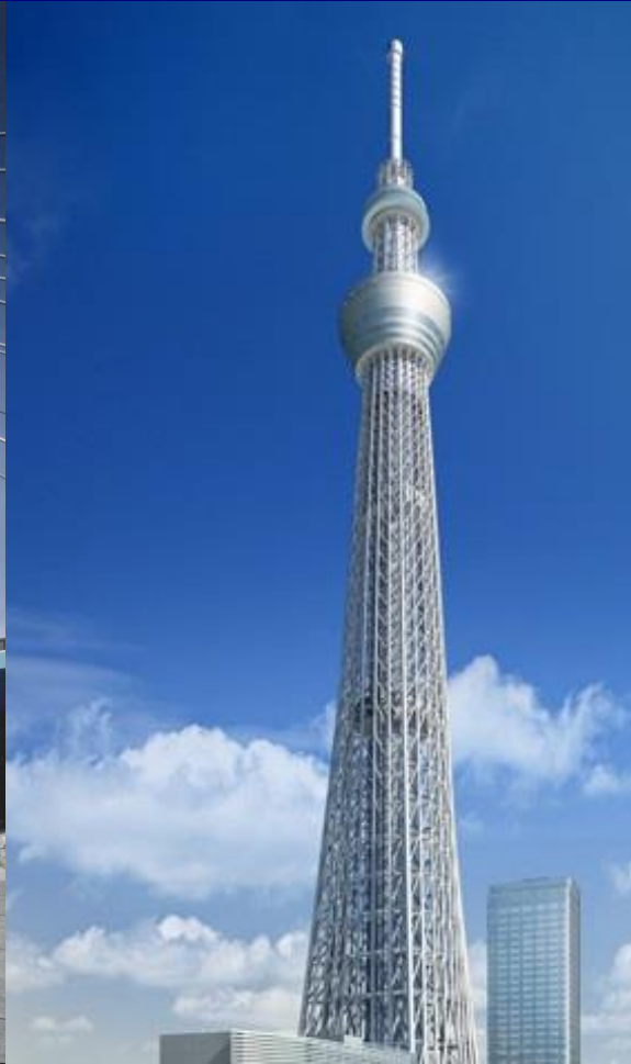
Steel Structure Fabrication
