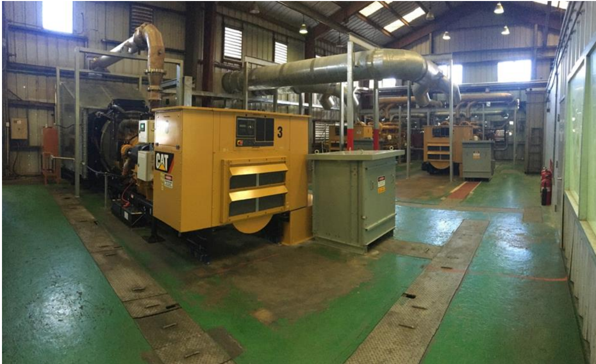
1 * 800 kw Cat Diesel genset
