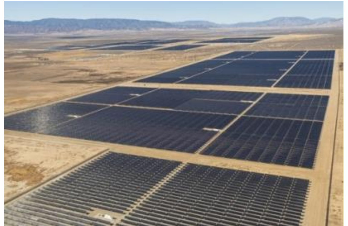
Astoria Project developed by Canadian Solar's subsidiary Recurrent Energy (100 MWac/131 MWp)
