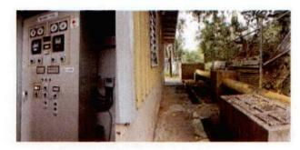
Flow monitoring system utilizes a magnetic flow converter that is installed along the transmission line and the monitor is situated insisde the pump house. The monitoring system needs to be calibrated.
