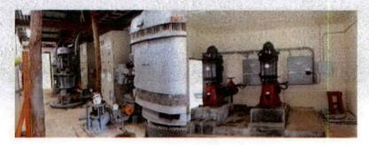
There are 6 units of transmission pumps and motors, 4units are 100hp vertical turbine pumps, only 3 are in operations, and 2units 150hp vertical turbine pumps that was installed last 2015, but 1 is not in operational due to electrical problems.
