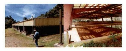
The sludge drying bed is housed in a steel structure where the steel are already corroded and the roofing system are leaking. The plumbing system of the drying beds are not functioning as per design. Instead of water from the silts being filtered and returning back to the wet well, it is now left to evaporate.
