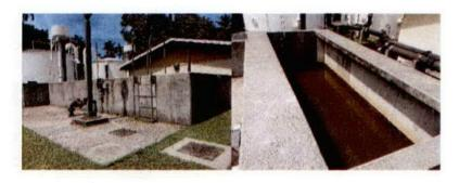
Wet well and backwash tank are incorporated in one structure. The backwas tank is much more deeper pit where the silts and sediments are collected. As planned, the backwash water from the gravity filters are collected by the backwash tank then pumped to the sludged drying bed, currently the sump pump is not operarional, thus the backwash water is directly released to the drain and sludged are manually removed.
