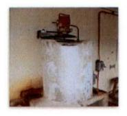
This Chlorine Agitator & tank was commissioned in late 1998. Tank has already been replaced, and the motor was replaced only once. At present, the condition for all components is very poor.
