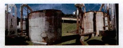
Gravity filters utilizing sand filter media. 5 units are commissioned, 3 units was serviced last 2015, changing sand filter media and other maintenance.
