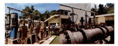
Originally, 4-20Hp vertical turbine pumps are installed, as of the present, 3units are operational at present.
