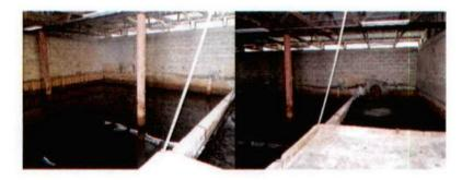
The main clearwell area is where the final treated water is stored prior to distribution, another small bypass clearwell is located beside this structure. Currently the the structural walls fo the maini clearwell are cracked and there is an ingress of ground water.
