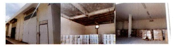
Chemical storage area is a concrete structure that is not properly ventilated. Due to corrosive effect of chlorine fumes, all the metal components inside the room are already corroded and damaged. Proper ventillation is needed.
