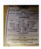
This emergency standby generator is being run since early 1990s, every time there is island power outage. It has been serviced by Caterpillar representative about ten years ago. This machine cannot function normally to power the two 150 Hp pumps. The engine/generator display module is completely not functioning.
