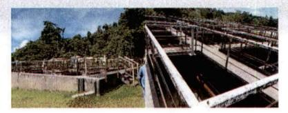
Due to the direct exposure to the elements, the fibers of the railings are exposed and are health hazzards.
