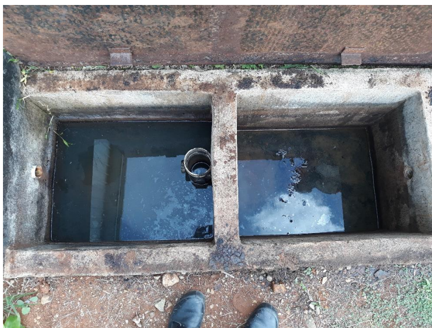
Figure 2 Interior 2 stage interceptor
