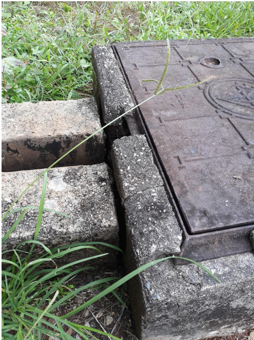
Figure 1 Inlet of Oil Interceptor
