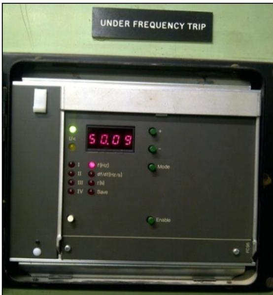
Figure 8 ABB FCN Frequency Relay Meiro Sub Station
