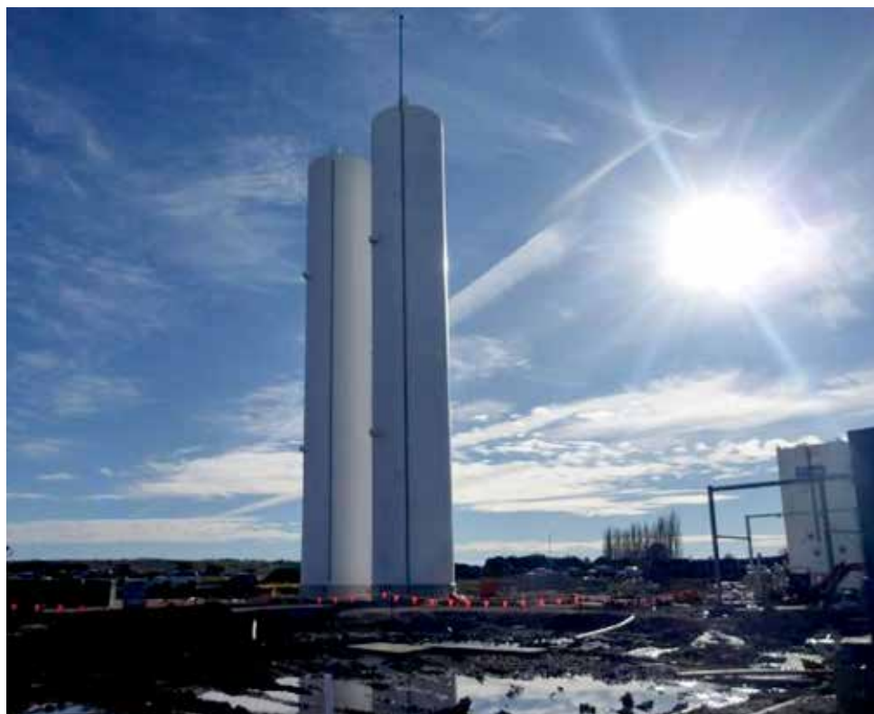
Figure 31. 300m 3 Cryogenic LNG Tank in Tasmania
