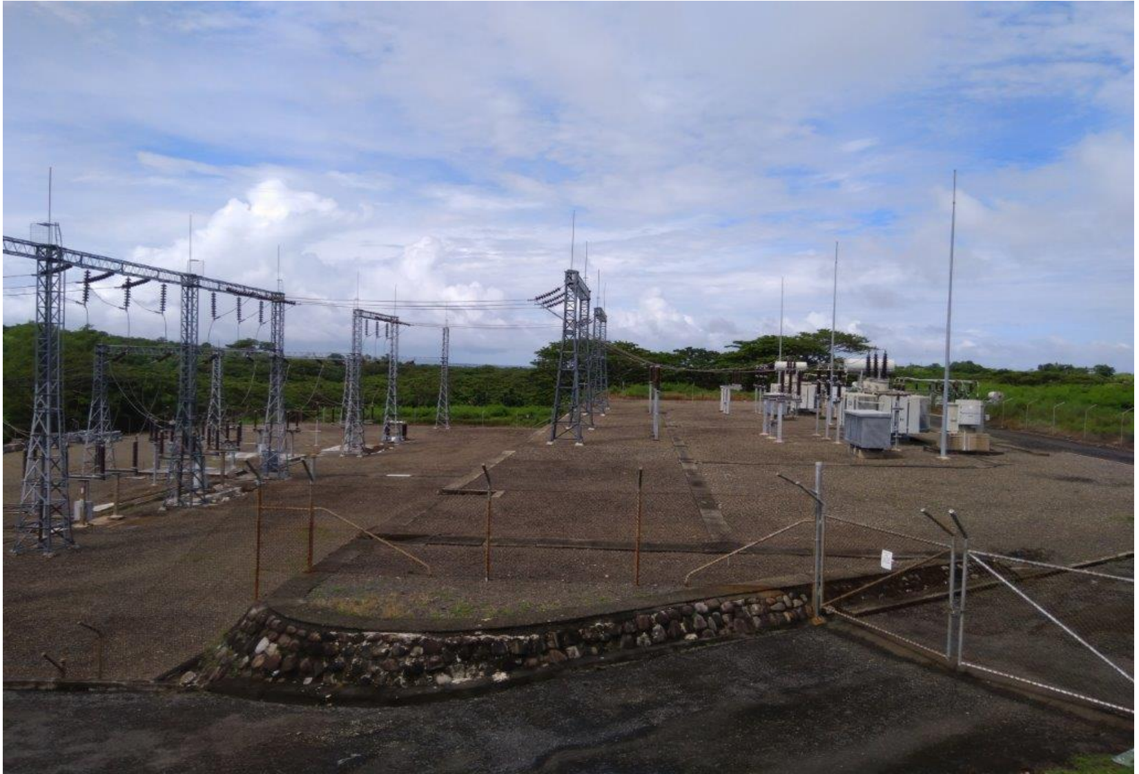
Vuda 132kV/33kV Zone Substation
