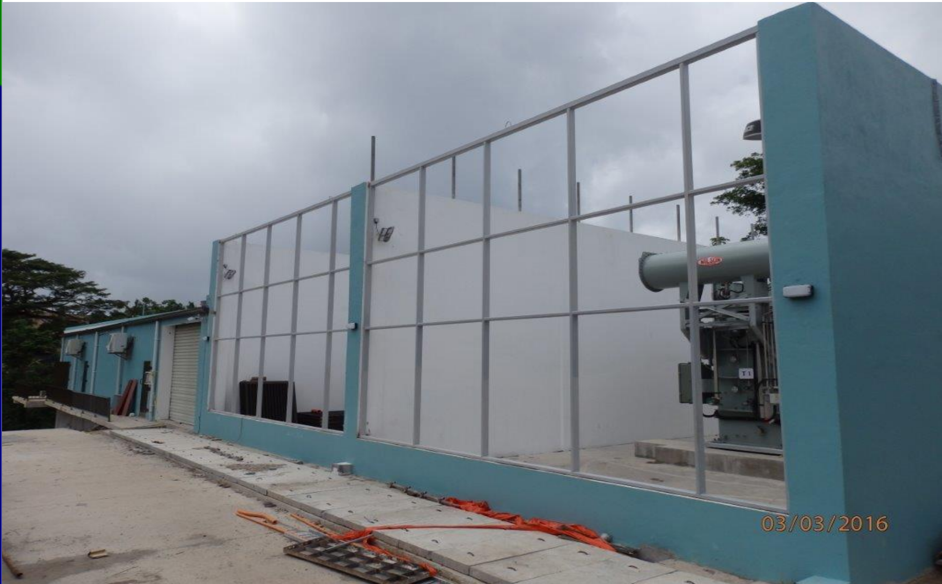
Knolly Street 33kV/11kV Zone Substation
