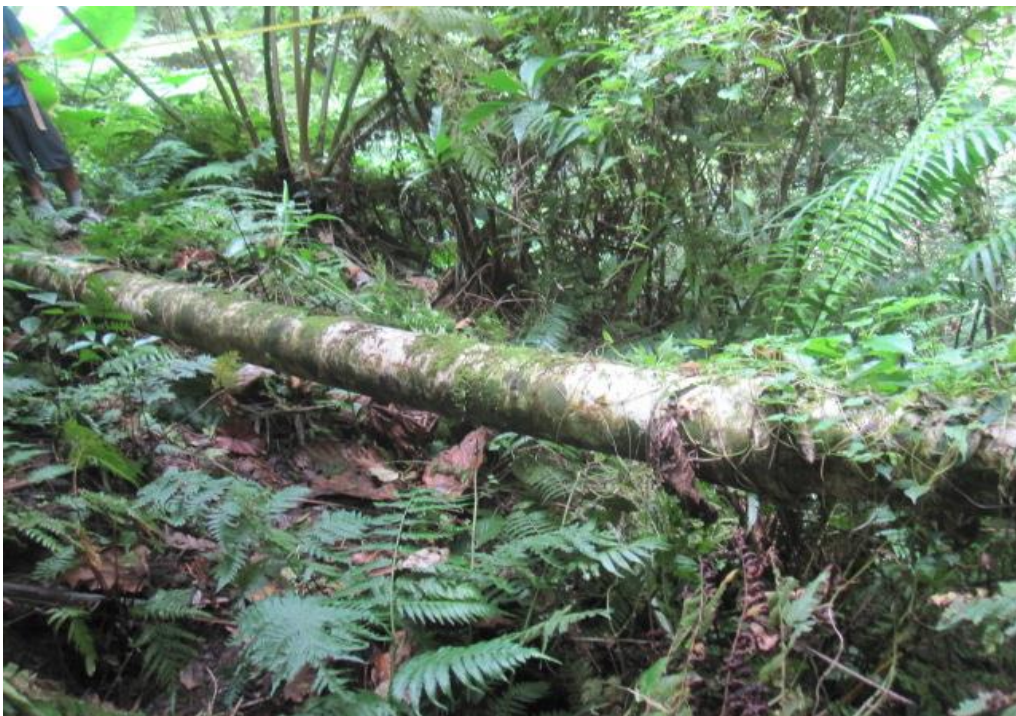
Photo 6: PVC pipe to be supported.
