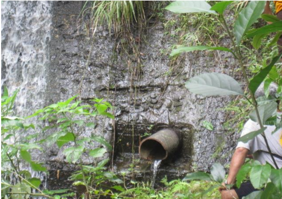
Photo 7: Drain pipe to be repaired.
