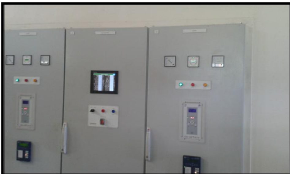
Figure 8: Taelefaga Plant's Existing Generator Control Panel
