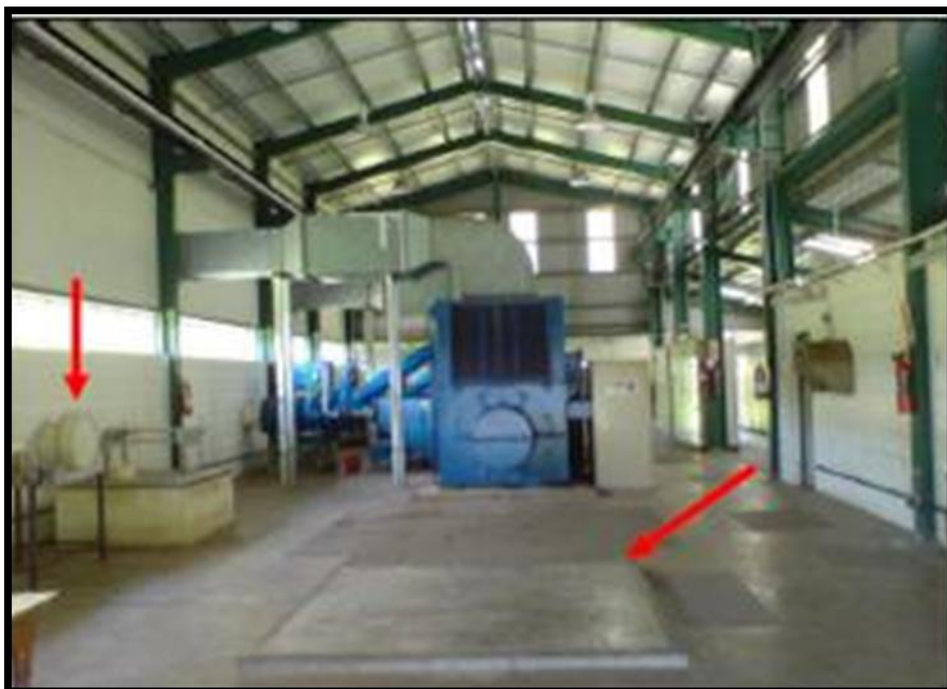
Figure 4: Generator No 1 is closer to this side of picture. Spare bay is for 3 rd Generator installed under a different contract.
