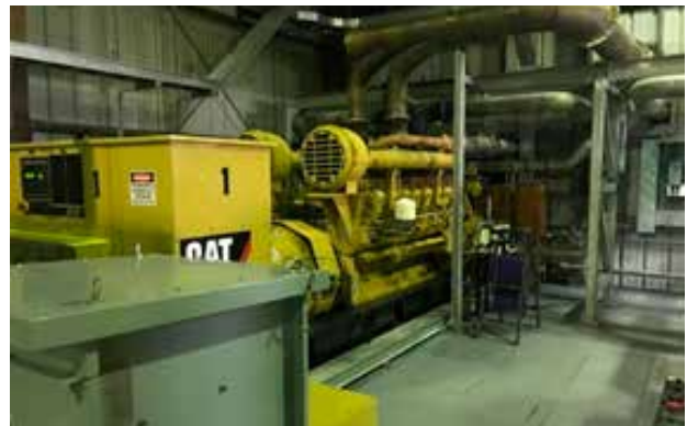
Automated and real-time high-speed diesel generators
