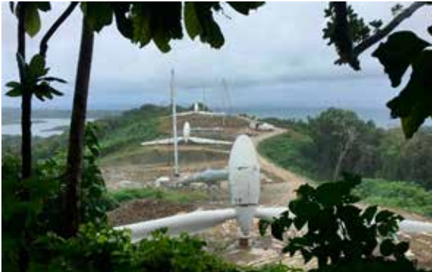
The three wind turbines secured on the ground
