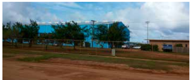
Solar PV rooftop installed in the Sports Complex
