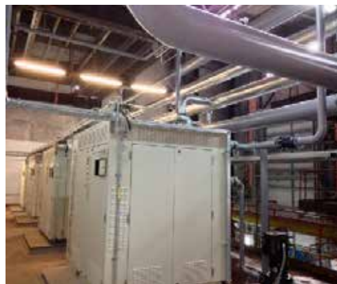
Figure 2. ElectraTherm recently installed ten Power+ Generator 4400s at a district heating plant in Slovakia.
