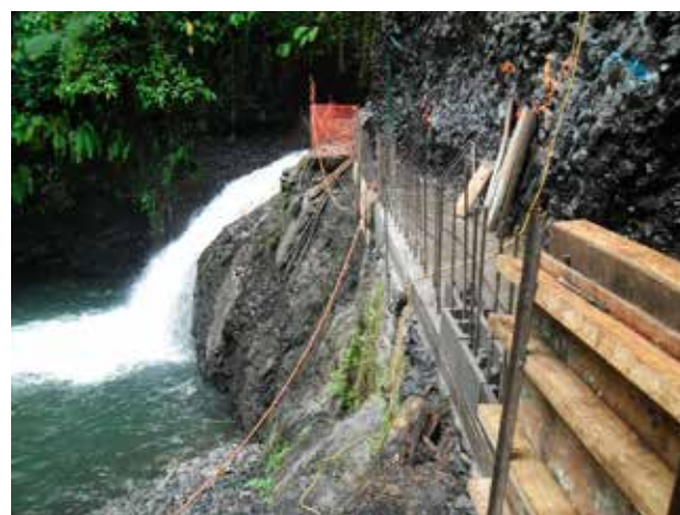
Clearing of the Samasoni Hydro Power Plant pond and the newly constructed Alaoa east intake
