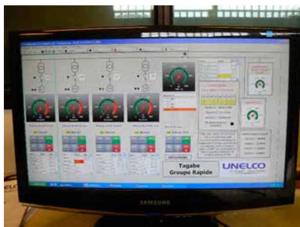
InteliMonitor SCADA screen for a four-set power station
