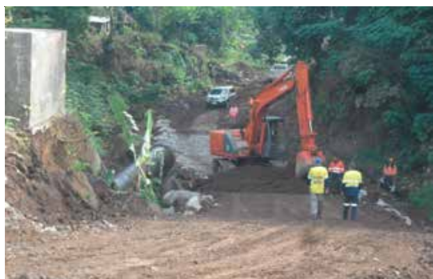
Civil works during construction and the laying of pipelines
