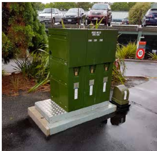
Halo solid ring main units are scalable. New modules and functionality can be added later to meet future requirements.
