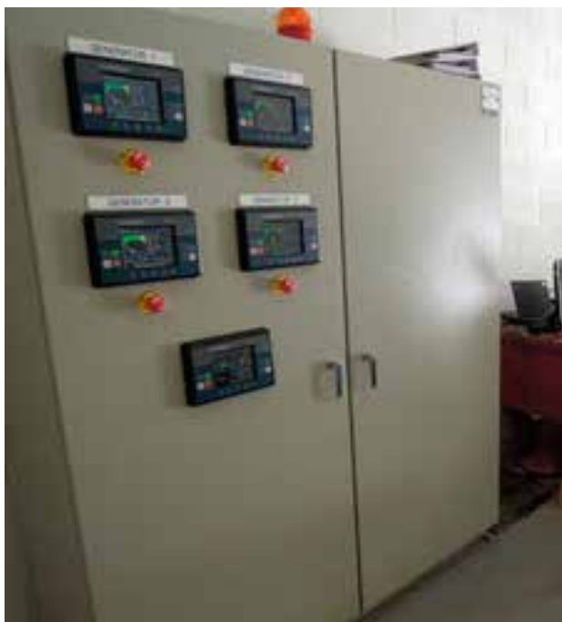
An automated control system for a four-set power station
