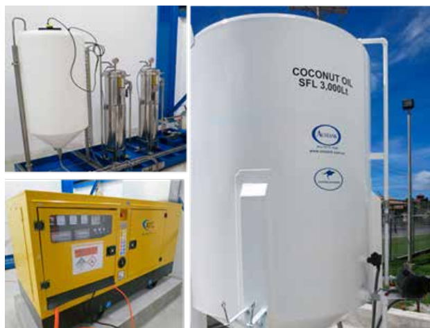
Image 2. The CNO generator and fuel tank
