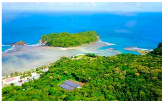
Ofu Solar PV Project
