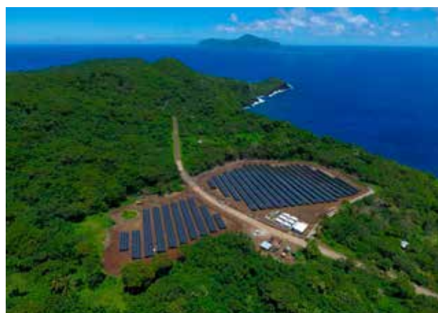
Ta'u Island Solar PV and Battery Storage System
