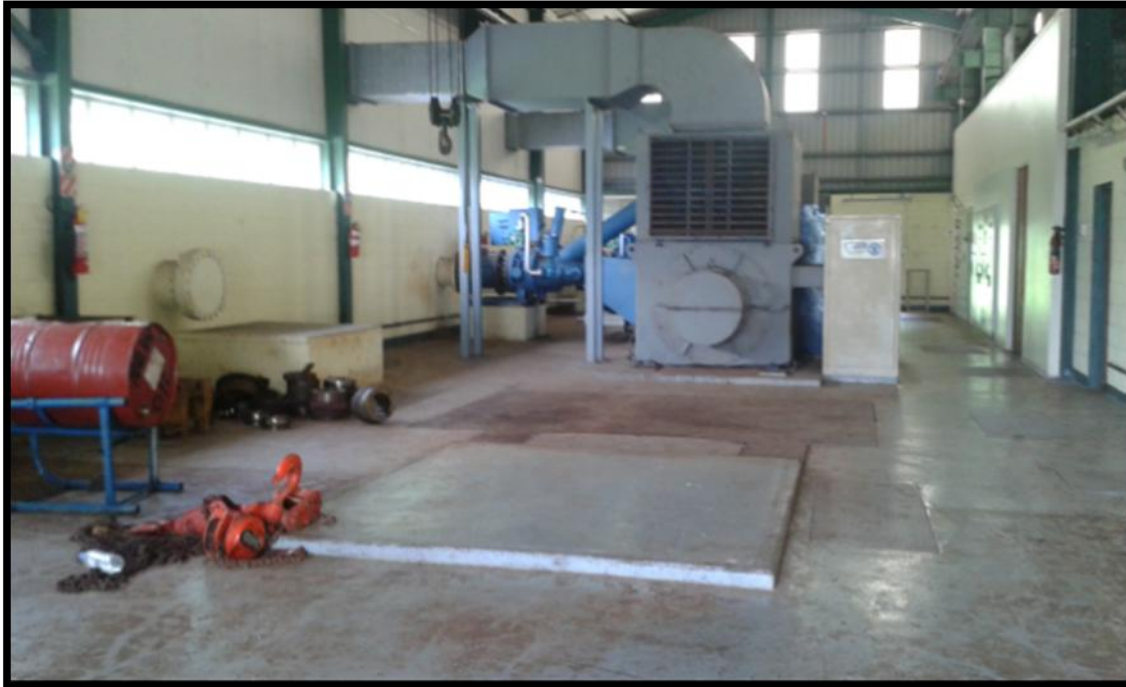
Figure 6: Third Taelefaga generator space
