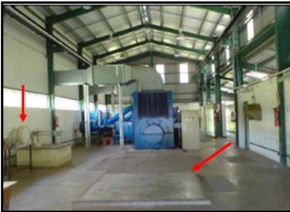
Figure 4: Space for third generator at Taelefaga power station.
