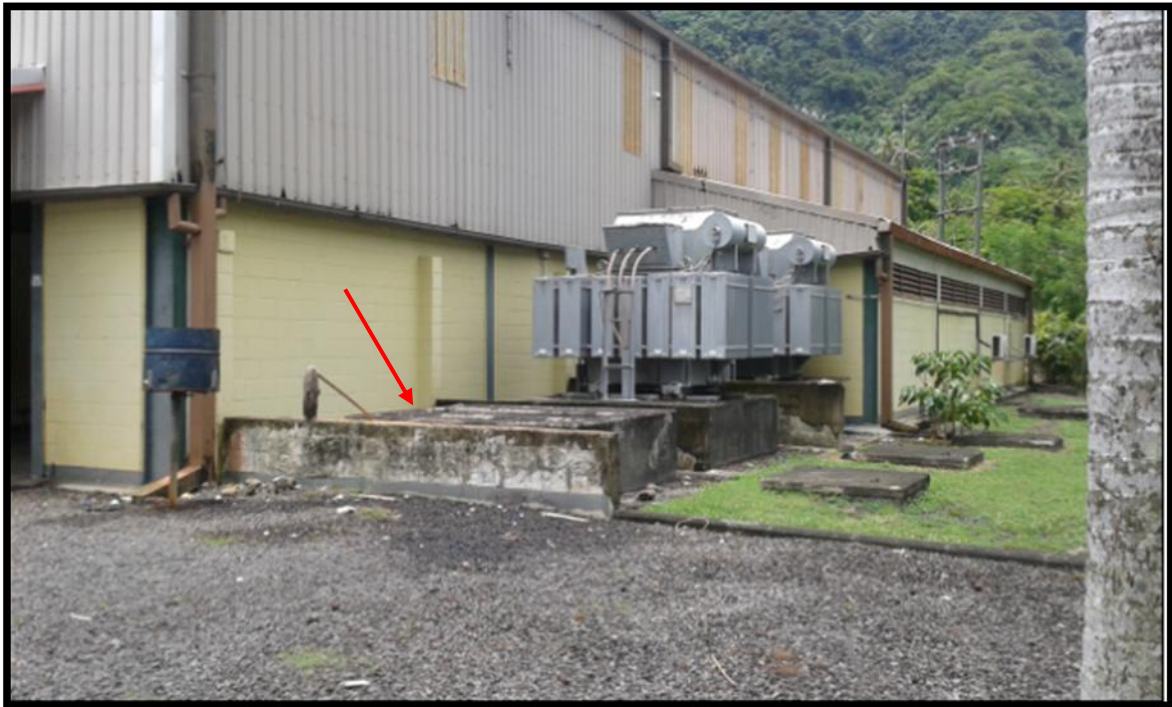
Figure 7: Taelefaga Station Step-Up Transformer pad for third generator
