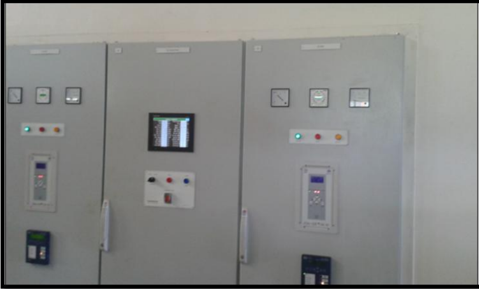
Figure 8: Taeléfaga's Control Panel
