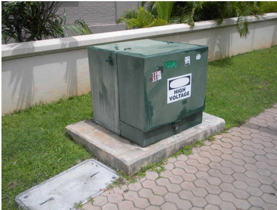
Exhibit 3-1: Pad-Mounted Transformer
